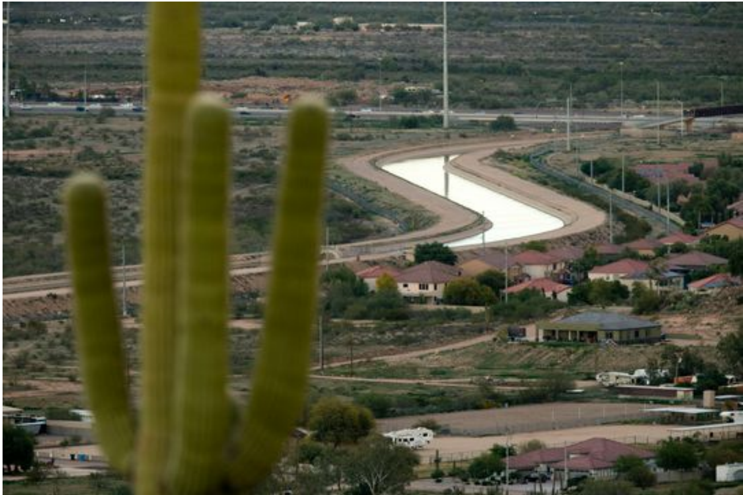
The CAP Canal winds through a neighborhood in Phoenix as seen from the Deem Hills Recreation Area on December 11, 2018. (Photo11: David Wallace/The Republic)
