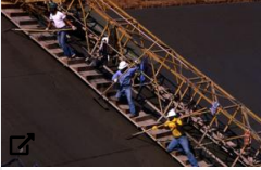
Photos: Central Arizona Project construction in 1973 Arizona Daily Star Jun 28, 2018
