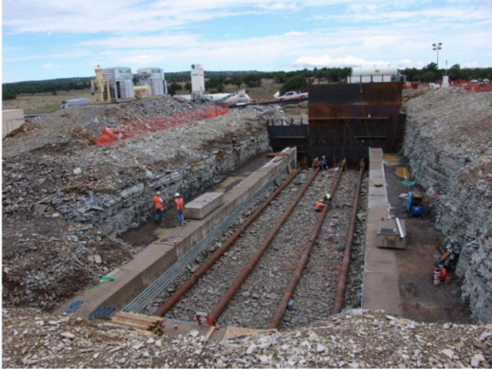
Red Leaf Resources has produced more than 300 barrels from its pilot capsule that tested ore from its oil shale mine in the Uinta Basin. This 2009 photo shows the capsule under construction on state land where Red Leaf heated kerogen-bearing ore to 725 degrees for seven months. Hot gas runs through the pipes and heats up the enclosed capsule like a convection oven.
