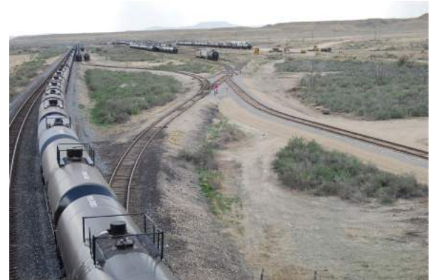
(Brian Maffly | Tribune file photo) The Price River Terminal in Wellington trans-loads from trucks to rail cars, opening a new path for Uinta Basin crude to reach out-of-state markets. Officials in a coalition of seven eastern Utah counties are hoping to link such facilities with oil- and gas producing sites using millions of dollars in federal mineral royalties.
