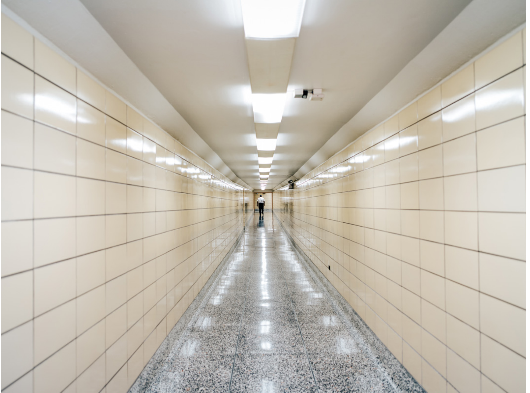
A hallway inside the Glen Canyon Dam.
