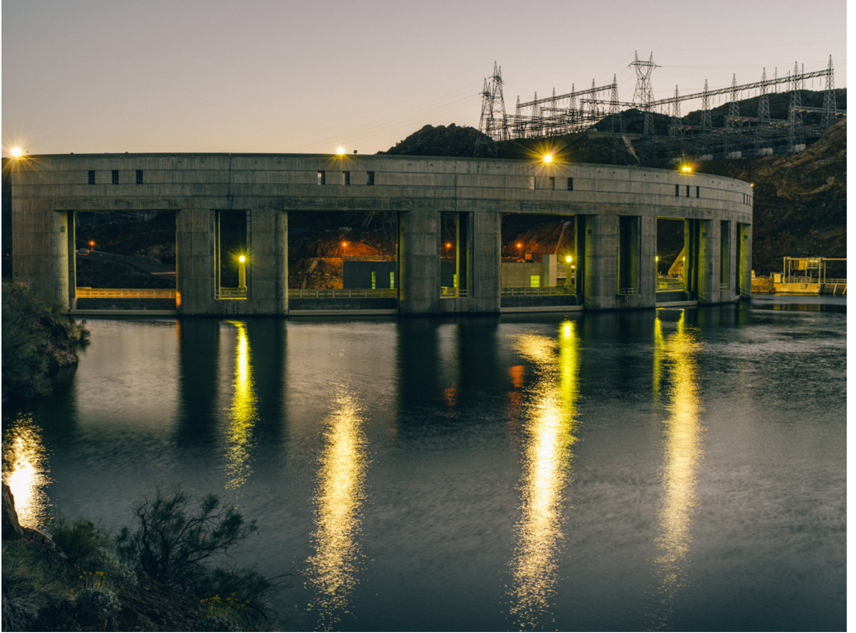
The Parker Dam on the border of California and Arizona. Said to be the "deepest dam in the world," with some 235 feet of it below the riverbed of the Colorado.
