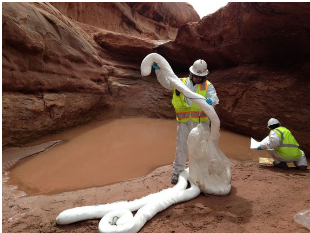
(Courtesy photo) | Bureau of Land Management Crews work to clean up damage from a leaking oil well in Salt Wash, about 12 miles southeast of Green River.
