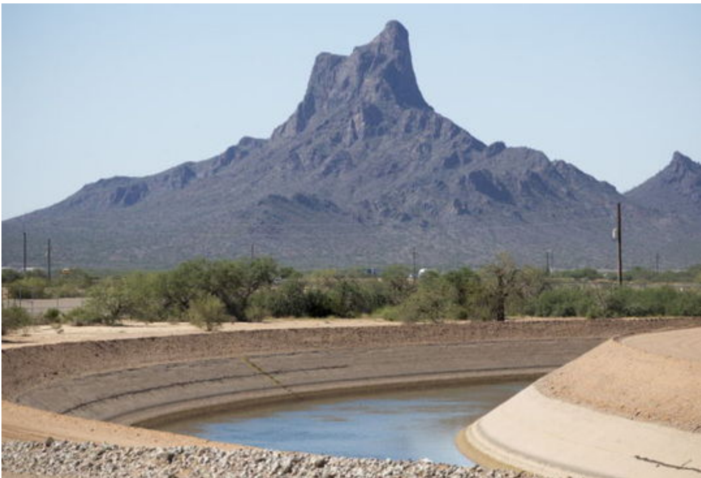
The Central Arizona Project delivers water to Tucson and Phoenix via canals like this one at Picacho Peak.
