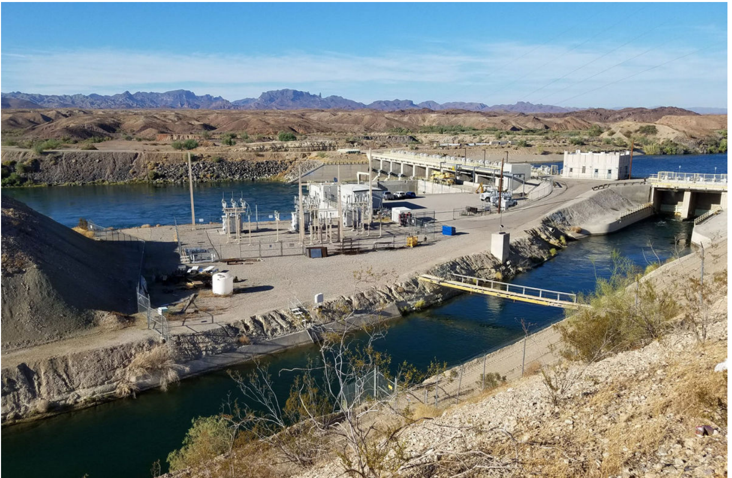
Headgate Rock Dam near Parker diverts Colorado River water onto Colorado River Indian Tribes farmland. The Colorado River and Lake Moovalya are in the background, with the main canal in the foreground.
