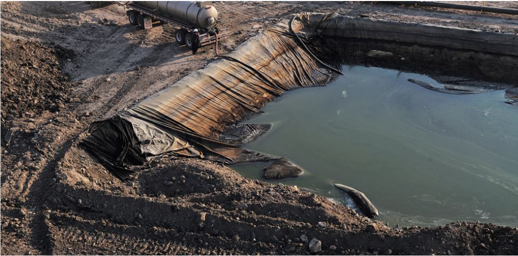
Fracking operations truck their liquid refuse to evaporation ponds, where it dissipates into the air. Marc Silver/The Filmmaker Fund
